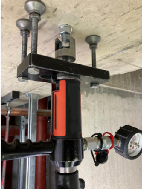
Tensile Load Testing for Anchors
